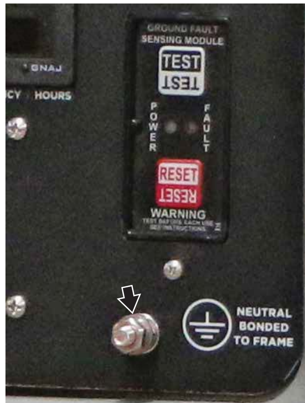
Figure 17 – Ground Terminal on the Control Panel
